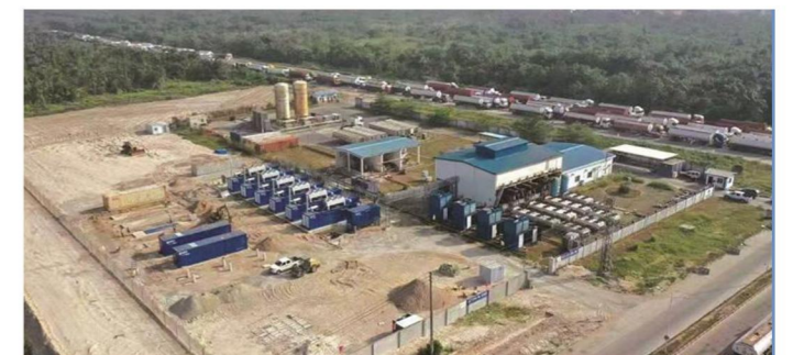
● Nigeria LEKKI CNG Power Plant
