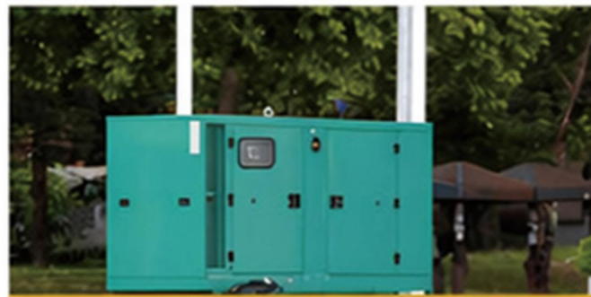
● Heilongjiang Harbin Municipal Project
