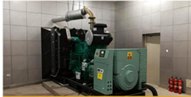
● Zhejiang Zhoushan Hospital Project
