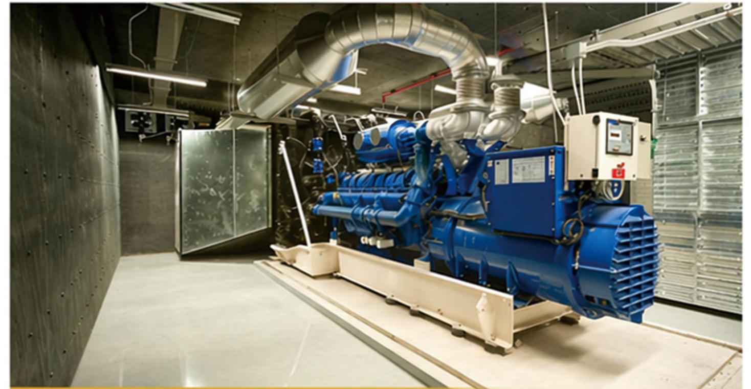
● China Petrochemical Jiangsu Branch Project
