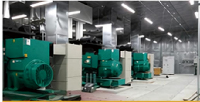
● Liaoning Anshan Mining Project
